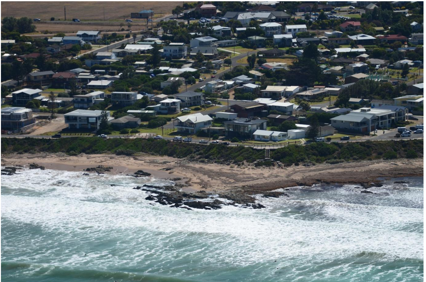
Narrow coastal reserves at Middleton Point (Coast Protection Board, March 2024)
