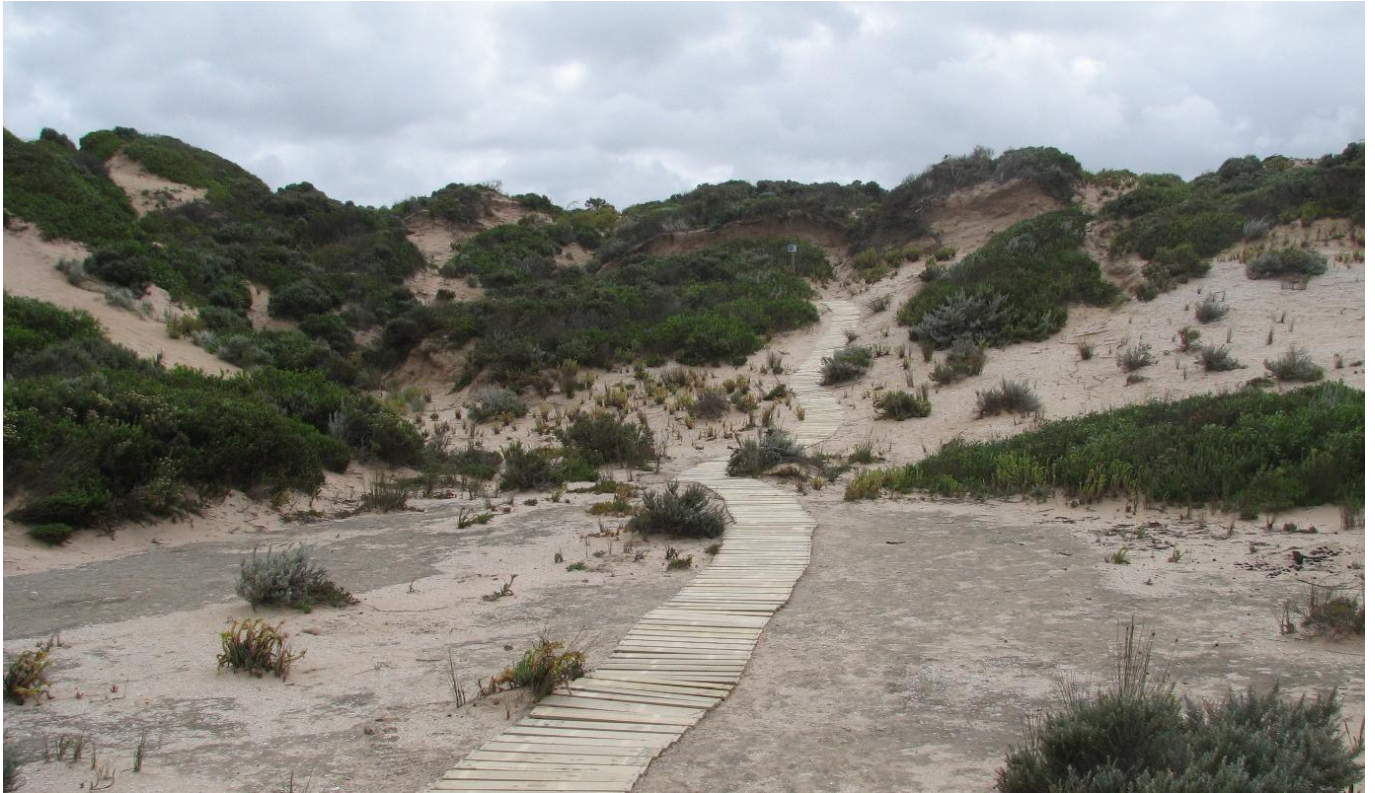
Access paths through the dunes using a dutch ladder construction method that can be lifted and replaced on the surface if buried by sand. Low impact and prevents erosion from multiple walking paths (B Simon)
