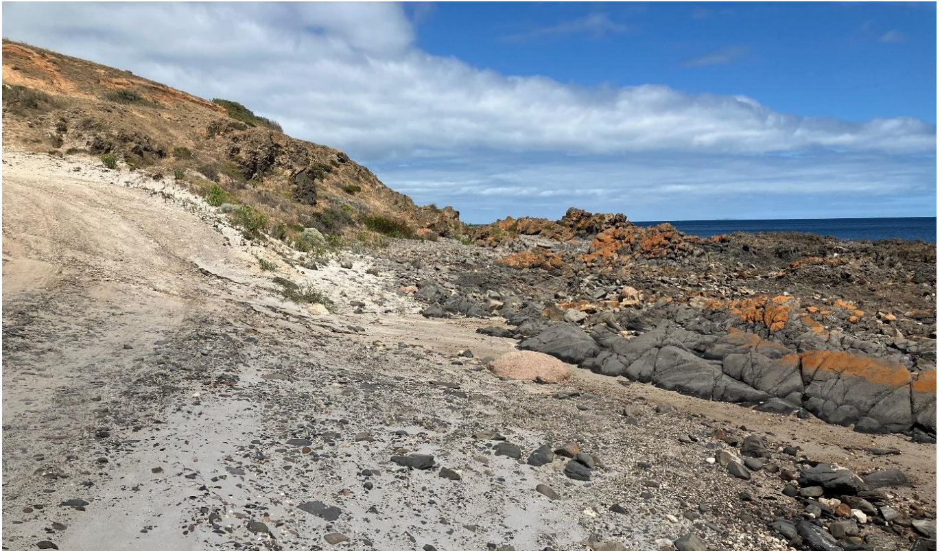
Erosion of vehicle access point and road surface from storm and surface water washing through onto and entering intertidal reef platform. (C Taylor)
