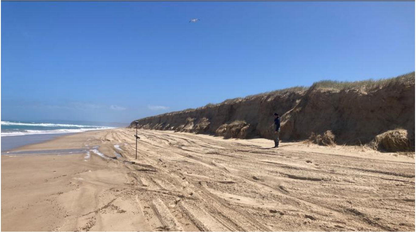
Beach Profile 615010 closest to the Murray Mouth showing erosion and scarping following cumulative impacts from 2025 storm events and vehicles tracks on beach (Coast Unit, DEW A Virag)
