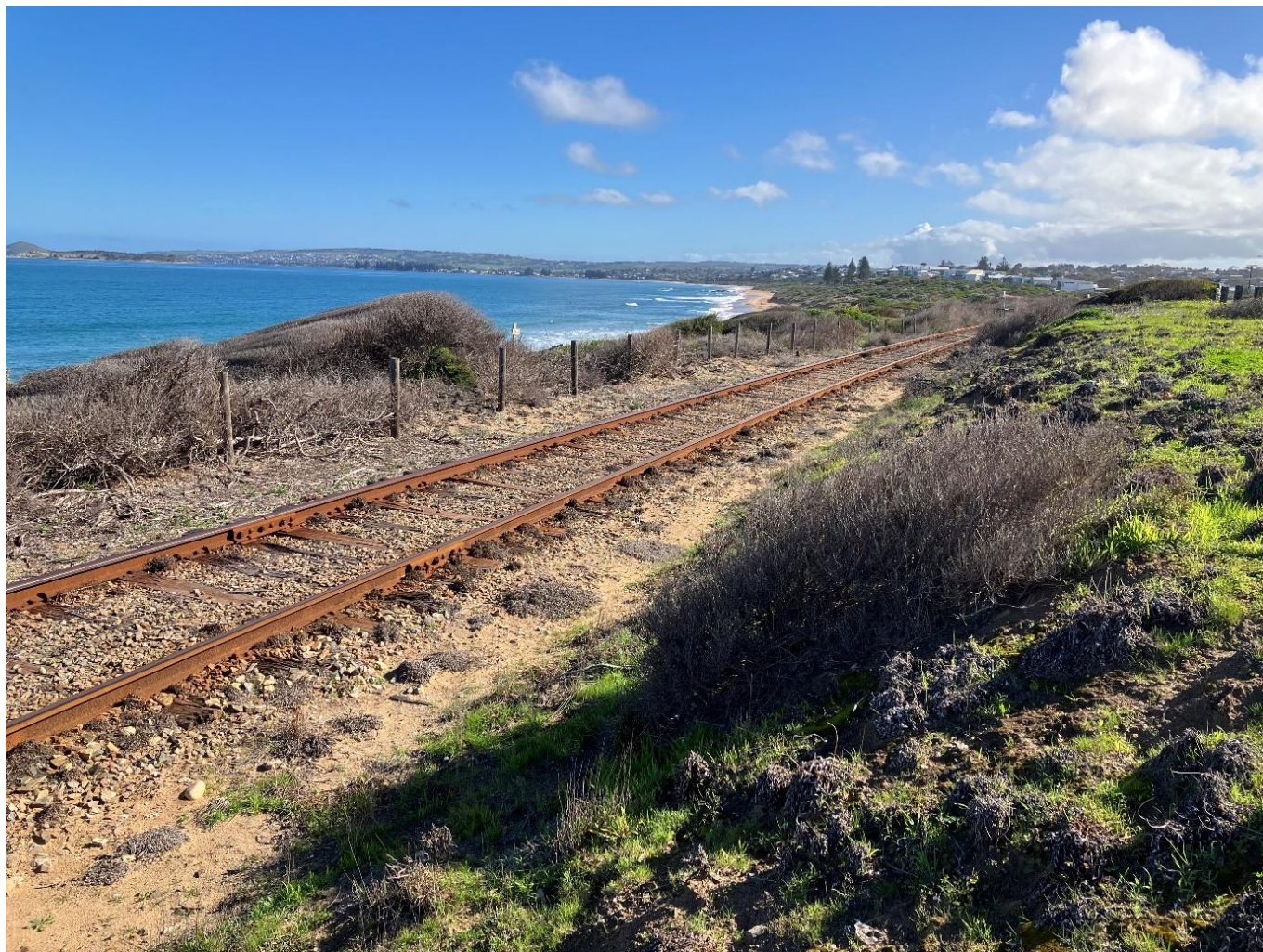
SteamRanger railway corridor, Watson's Gap (C Taylor)
