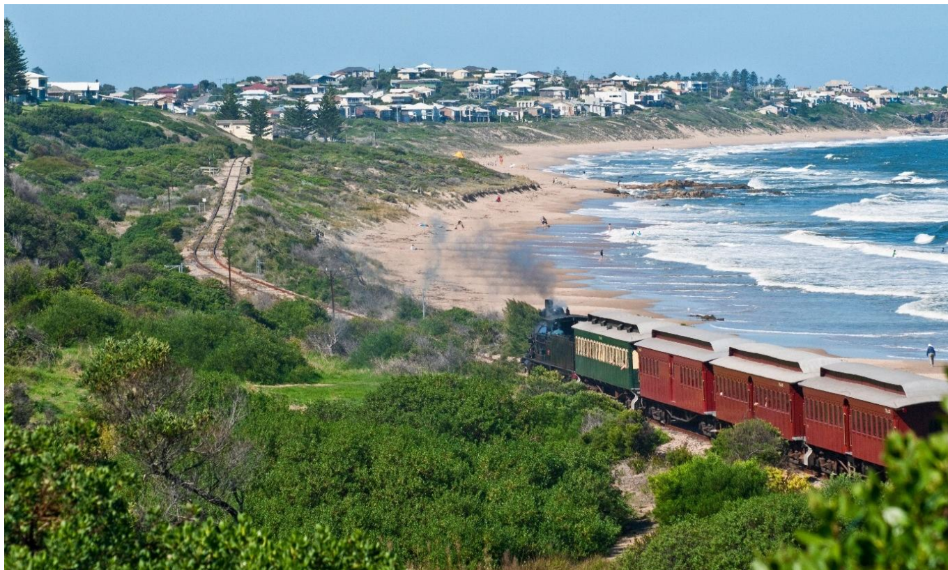
SteamRanger Heritage Railway corridor that sits atop of the dunes from Victor Harbor to Port Elliot (Graham Scheer)
