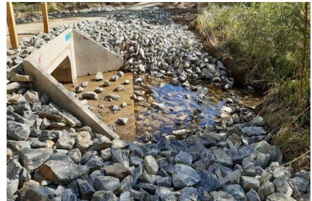
Figures 5 and 6: Cross-sectional diagram of fish passage dimensional requirements and a finished culvert base with secured rock to increase water turbulence for fish.
