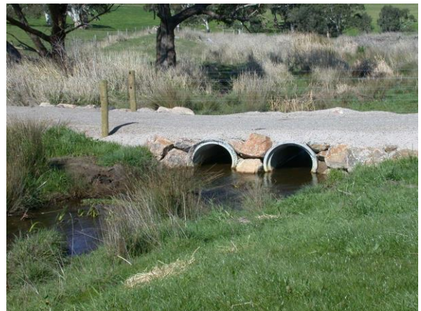
Figures 1 and 2: To the left is a dual boxed culvert and to the right is a dual piped culvert.
