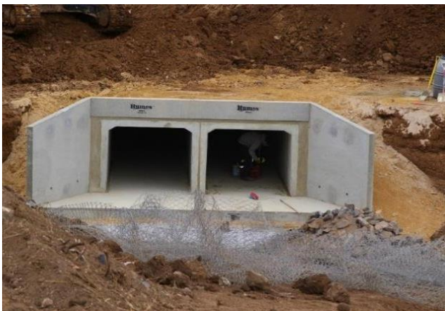
Figures 1 and 2: To the left is a dual boxed culvert and to the right is a dual piped culvert.
